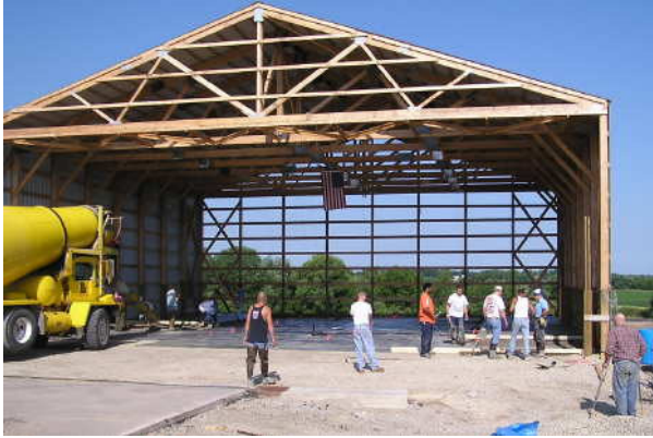
The crew worked on both sides of the hangar at once.
